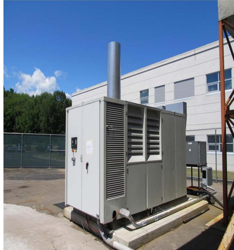
Figure 1: Newly Redesigned Microturbine
